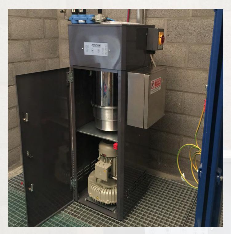
Every exhauster prevents the creation of static electricity, the motor overheating and others tricks. All ATEX exhausters of the wide STUCCHI range respects and goes beyond the security qualification imposed by the legislation, being always equipped with certified ATEX motors by the constructor.
