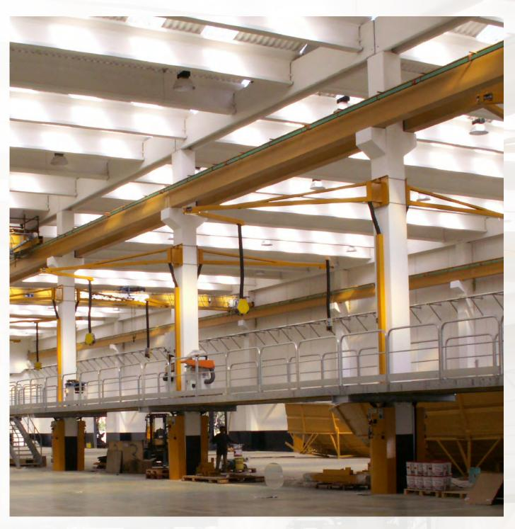
Articulated arms are available in three different measures B5 (5 m) e B6 (6 m) (if requested also 7 m). with this solution it's possible to remove the obstacle of electric cables, compressed air tubes and suction tubes.
